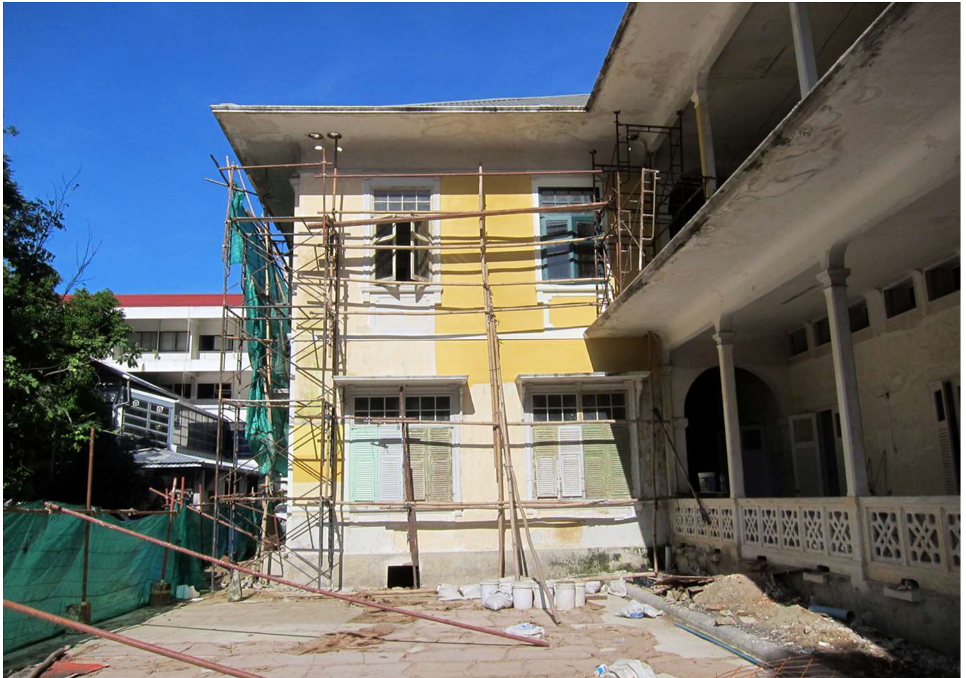
Paint test at Suthathip Ward during restoration
